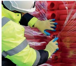
The plastic wrap is easily removed by carefully running a knife through the shrink wrap material.
