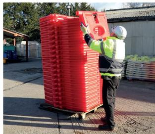
Carefully hold the barrier with one hand either side and ease the barrier down until below chest height.
